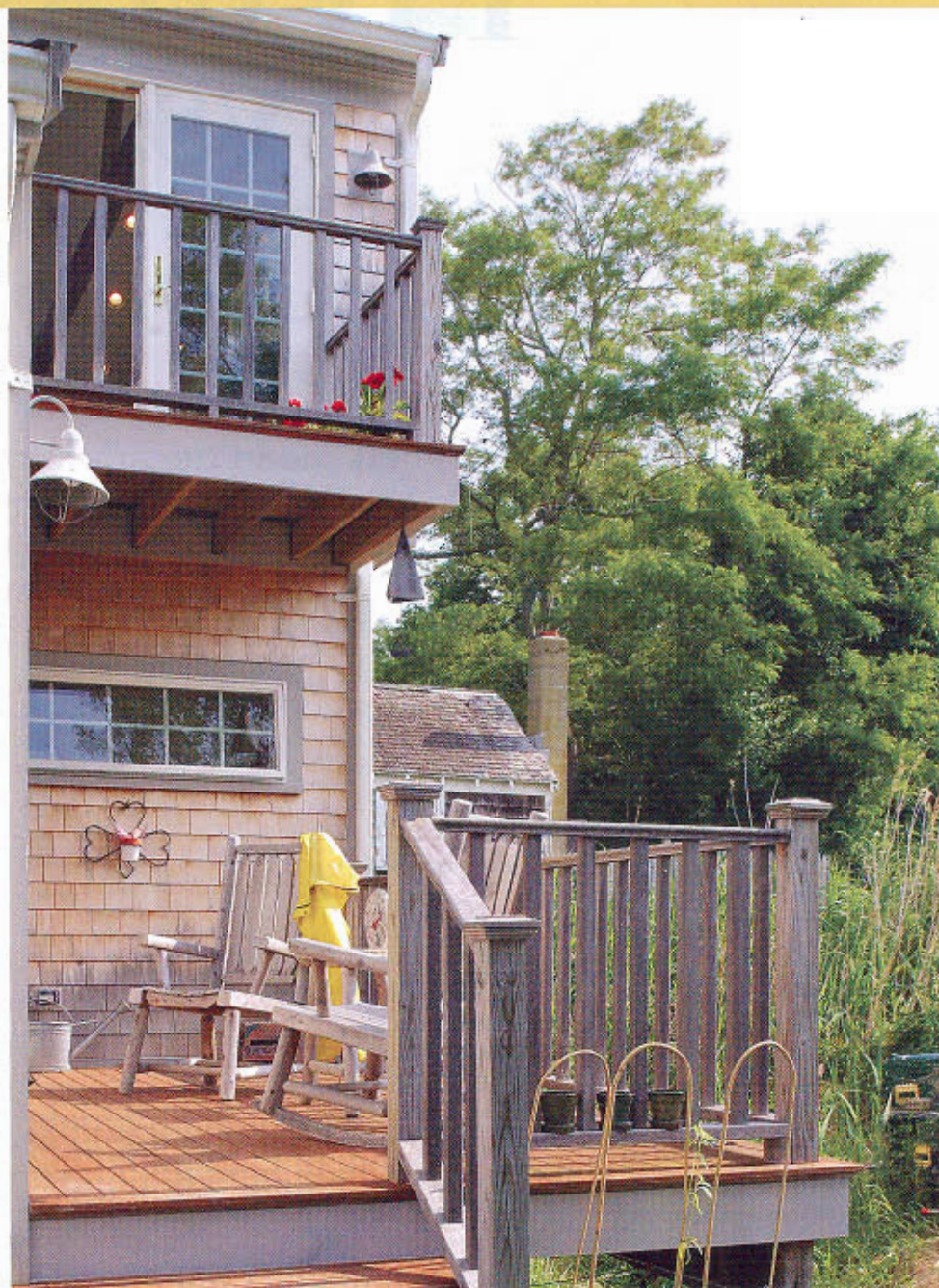
Decks complete the plan. The only additions to the existing footprint that were allowed are a second-floor balcony and a first-floor deck. Photo taken at E on floor plan.
